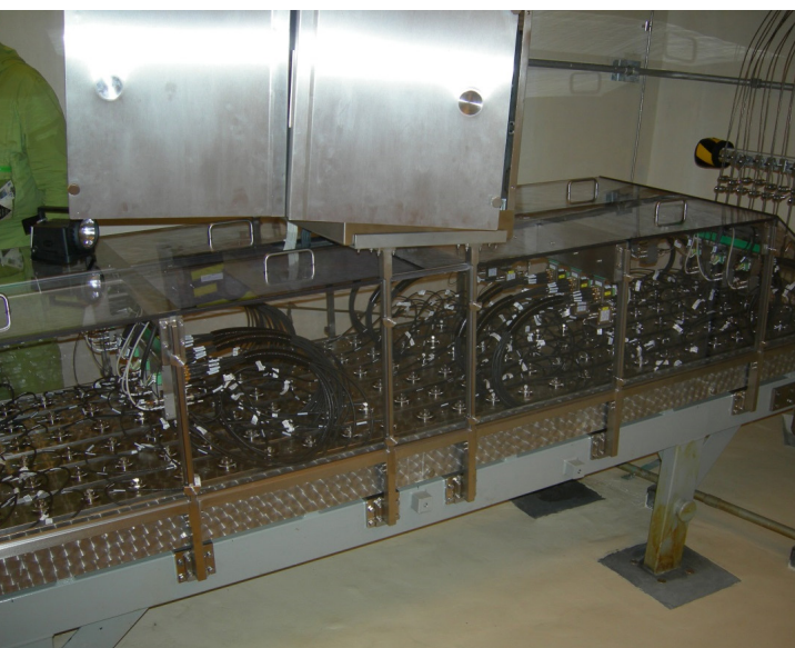
Trillo nuclear power plant neumobolas system
