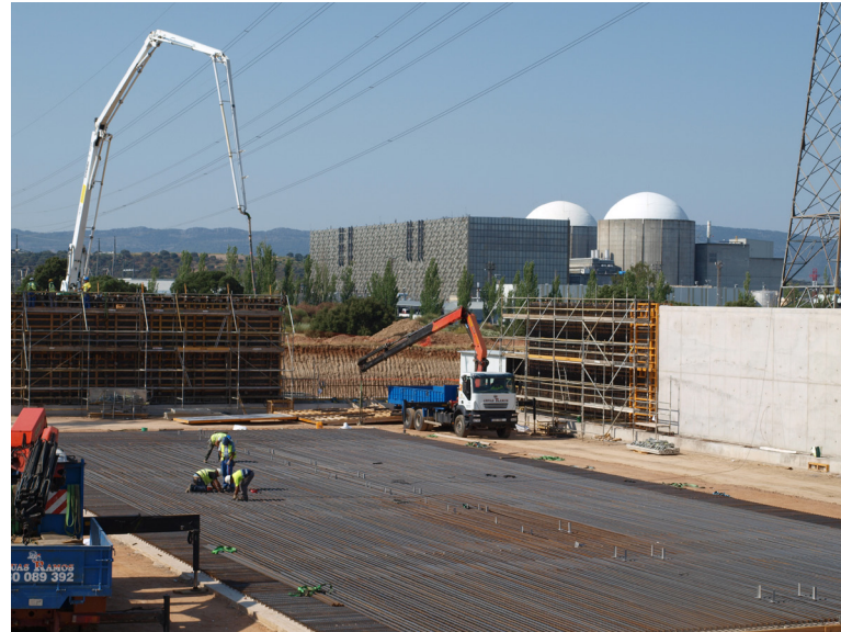
ISFSI: current status of works
